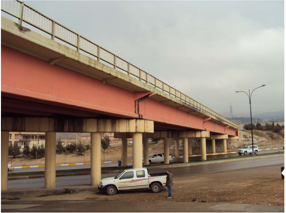
General state of the bridge looking north
